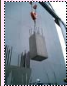
柱の吊りこみ
