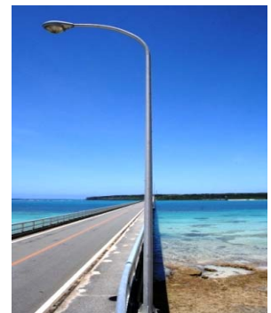
[宮古島来間大橋]
